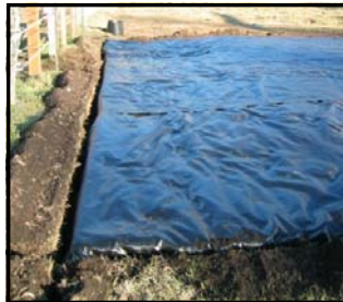
Geotextile fabric installed on bare ground and tucked into trench.
