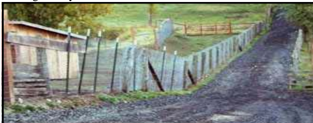
This lane, used to move cattle from their feeding area to their winter sacrifice pasture, was protected from mud by installing geotextile fabric and crushed gravel.
