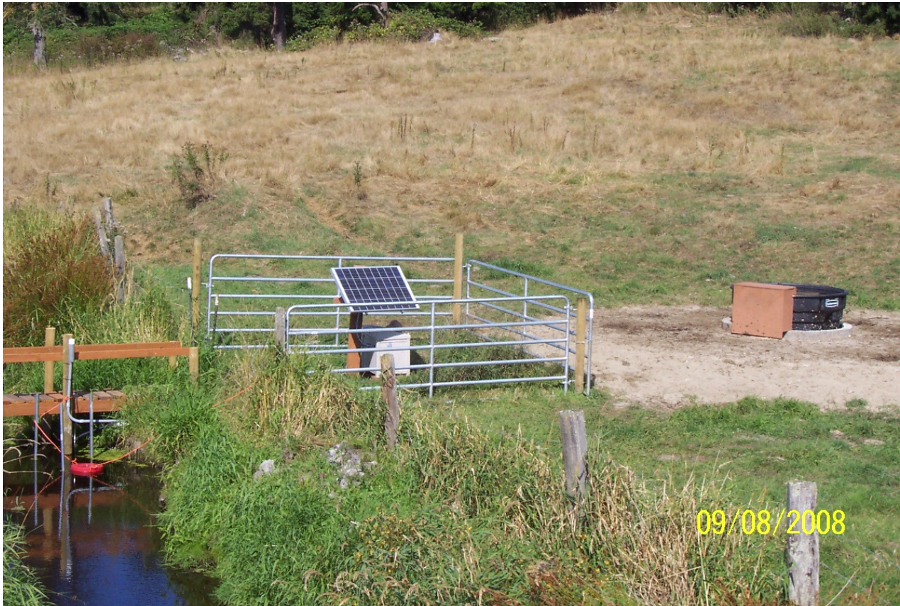
SOLAR POWERED LIVESTOCK WATER SYSTEM Chimacum Watershed
