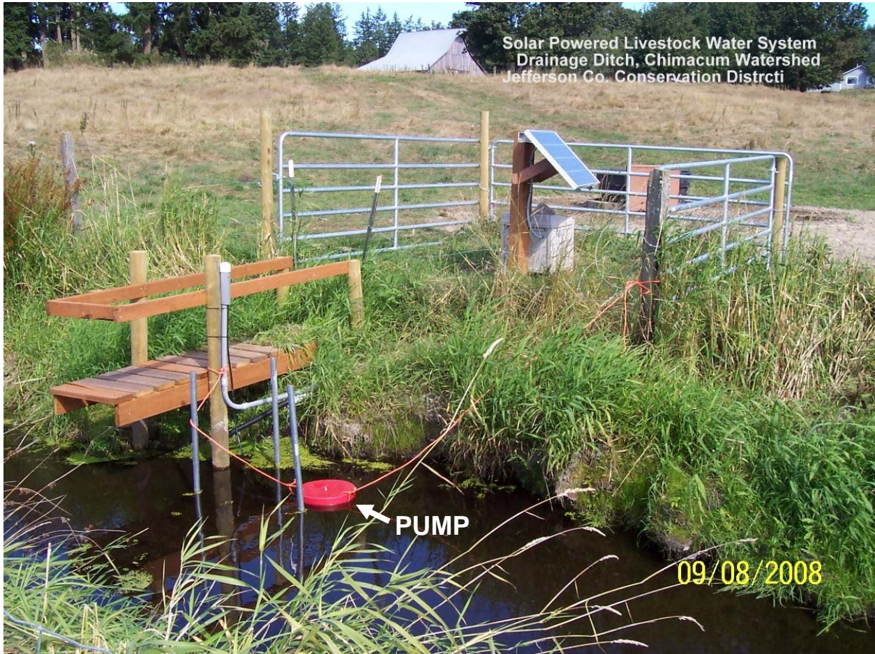
SOLAR POWERED LIVESTOCK WATER SYSTEM Chimacum Watershed
