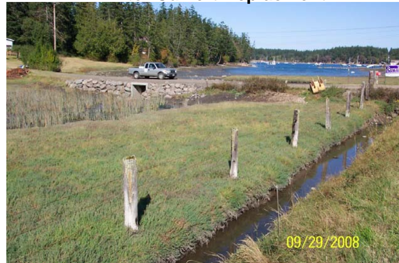
After Culvert Replacement
