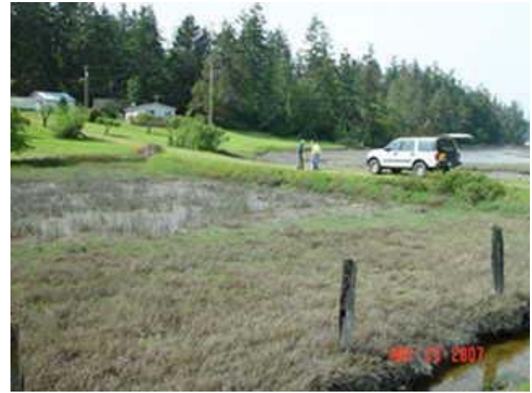
Before Culvert Replacement
