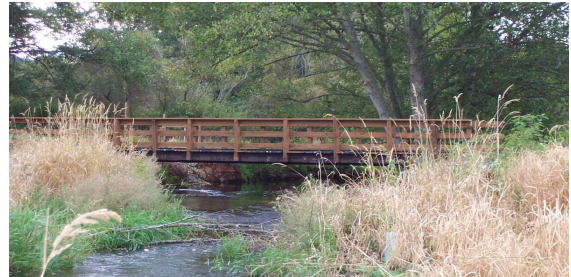
Newly constructed Spring Rain Farm Bridge
