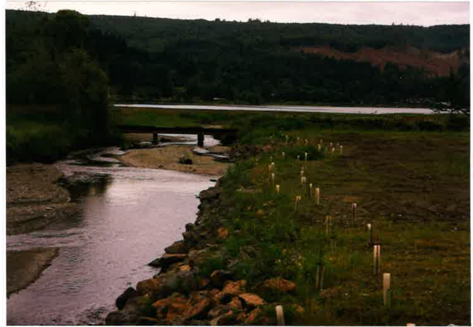
Downstream view from SR 20 bridge showing planted trees
