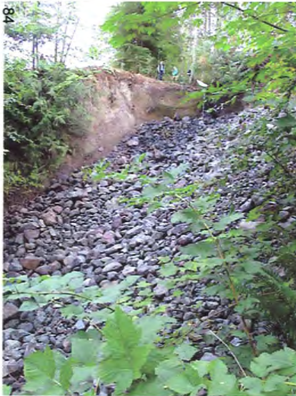
Figure 31. In August 2002, 1000 cubic yards of rock were placed in the gully which Houck Creek eroded when it was re-routed in the 1960's. A half-round culvert was placed at the top to prevent head-cutting.
