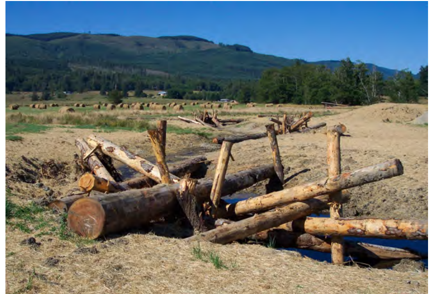
The new channel is ready for water!
