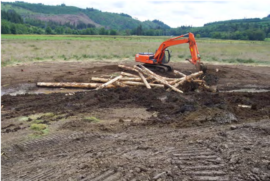
Large woody debris is placed in the channel.
