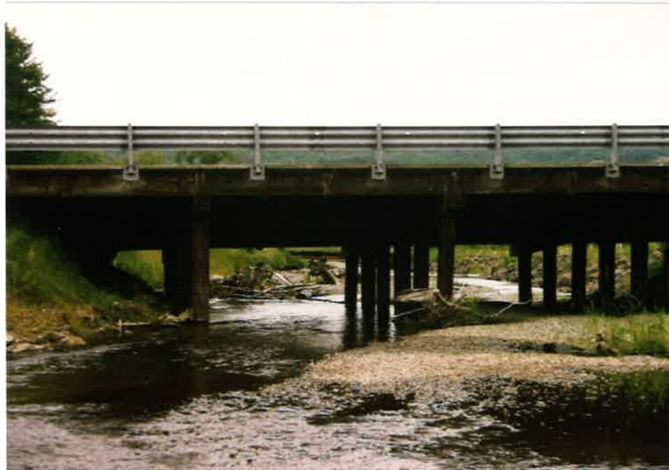
Downstream view from above SR 20 bridge Snow Creek
