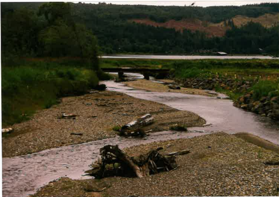
Downstream view from SR 20 bridge of widened stream channel
