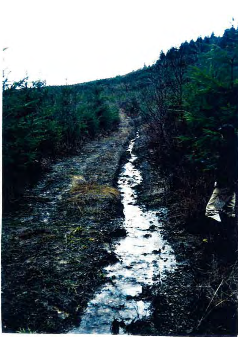
Figure 35. Eroded logging road and slope failure occurring in the upper Snow Creek Watershed (Sec 10, T28N, R2W) between stations SNO/4.4 (Snow Creek Ranch) and station SNO/7.0 (Snow Creek Road). Photographs taken in January 1995.
