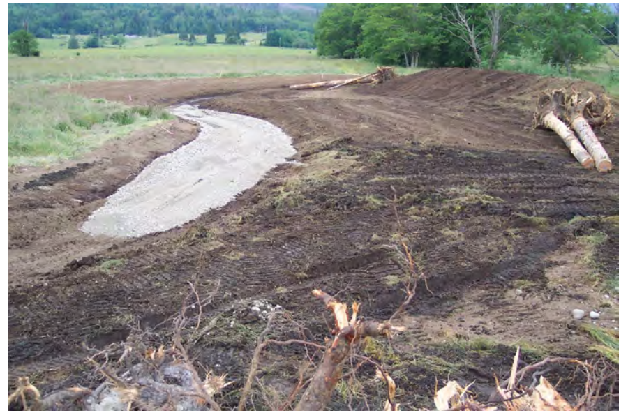
Gravel is added to the channel.
