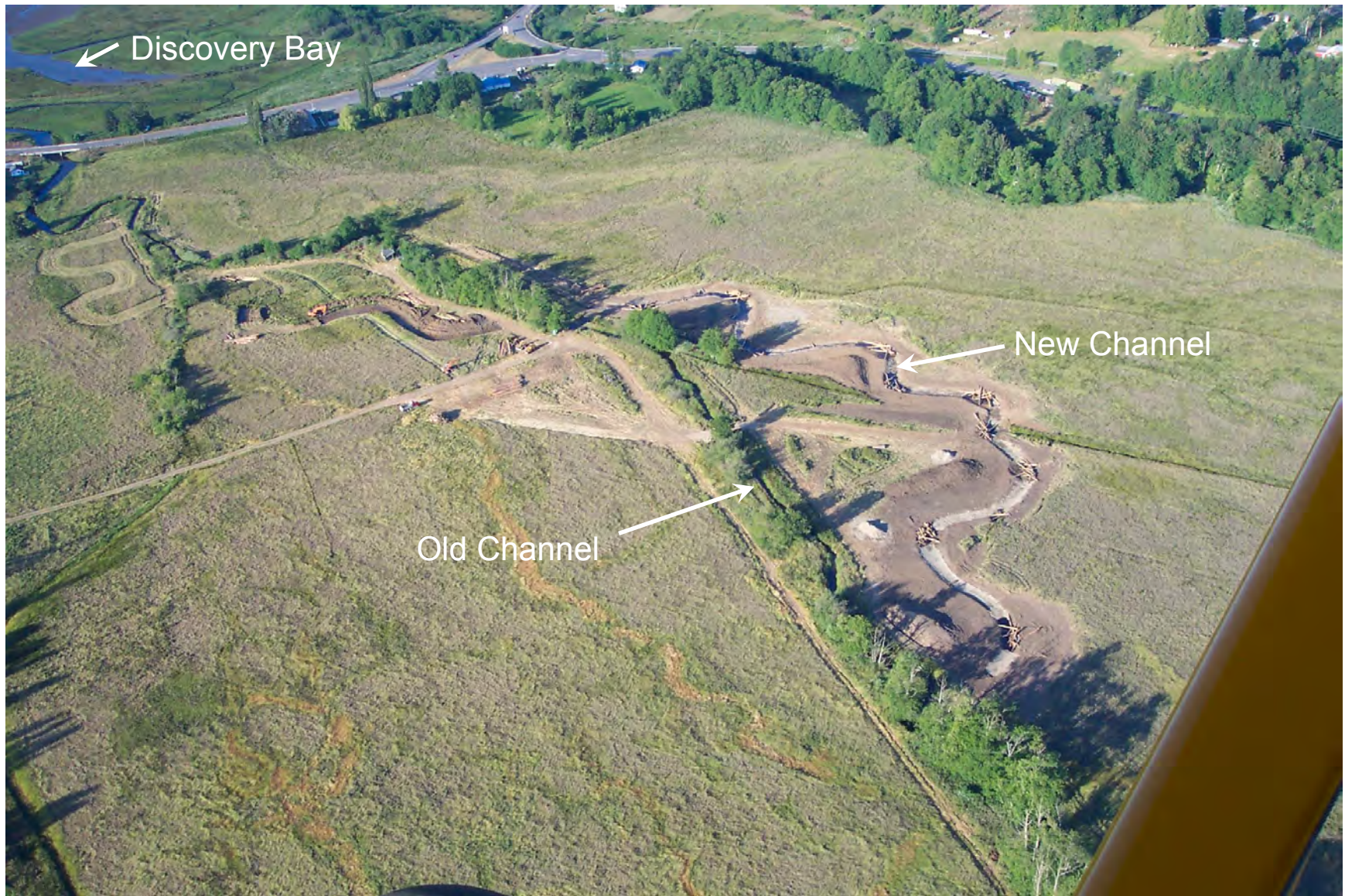
Figure 21. Aerial photo showing Salmon Creek's new channel constructed in 2003.
