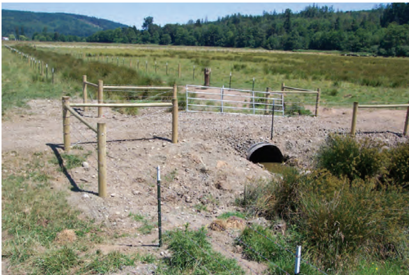
Uncas Valley ditch fencing and livestock crossing
