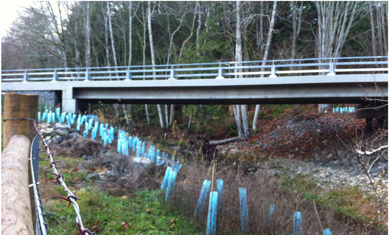
Wally Bowman Bridge on West Uncas Road was completed just in time for the 2019 Summer Chum run on Salmon Creek . Prior to this, it was necessary to place sand bags at the drop below the culvert to allow the Chum to pass upstream.
