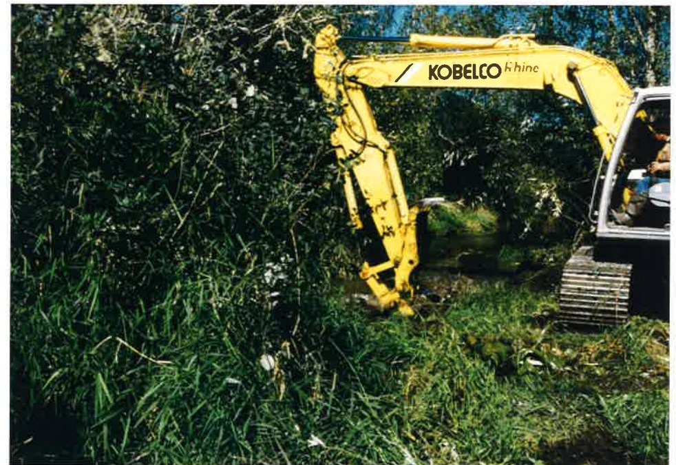
Sept. 1996--Channel being cleared by excavator
