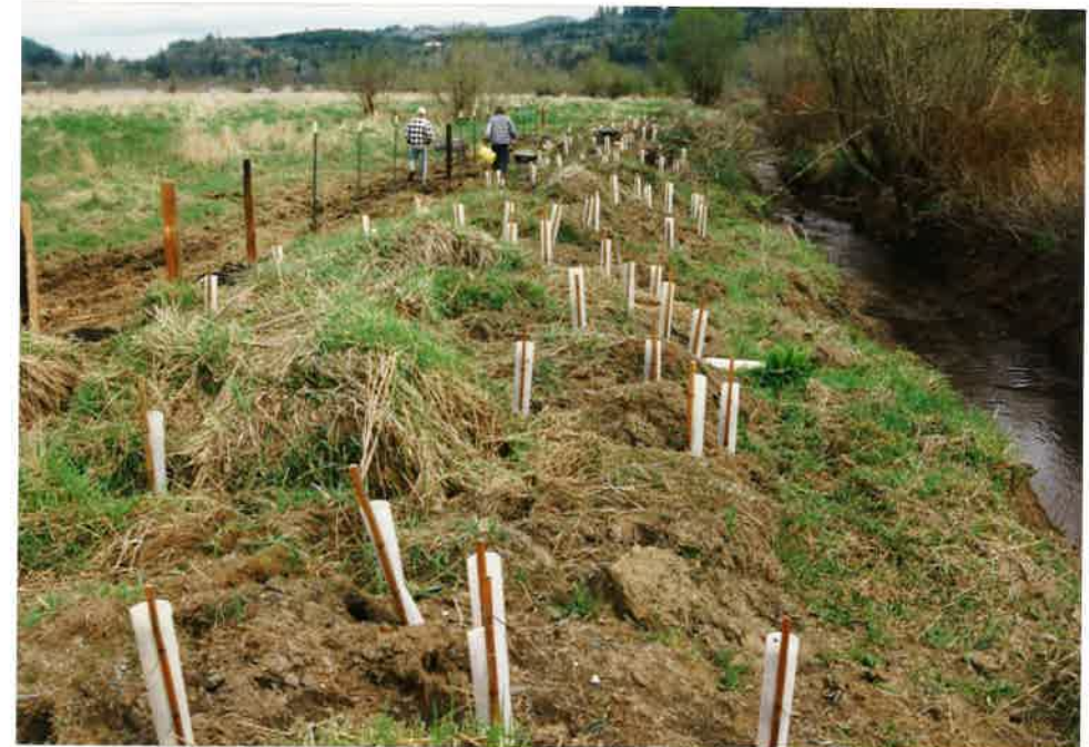
April 1997--Trees planted and fence under construction
