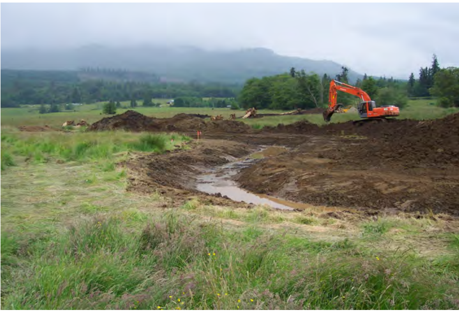
A new channel is excavated.
