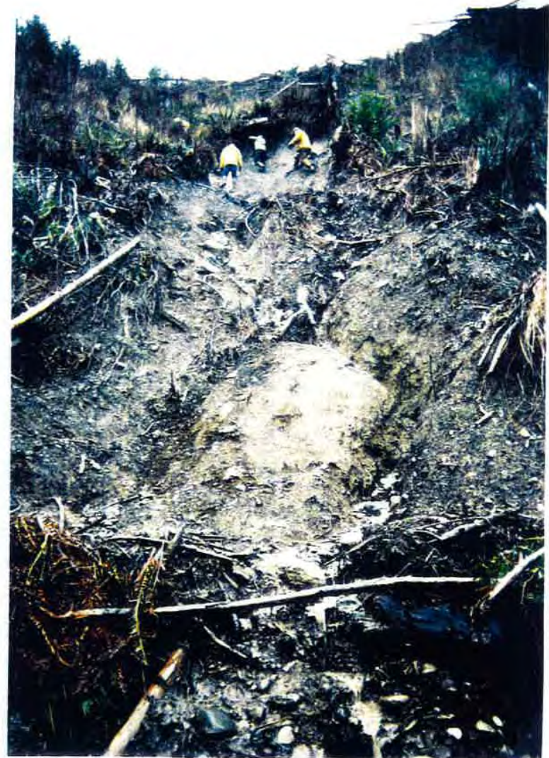
Figure 35. Eroded logging road and slope failure occurring in the upper Snow Creek Watershed (Sec 10, T28N, R2W) between stations SNO/4.4 (Snow Creek Ranch) and station SNO/7.0 (Snow Creek Road). Photographs taken in January 1995.
