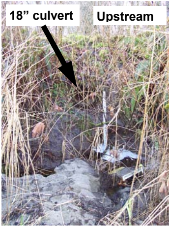
Hannan Culvert Removal Project, Swansonville Cr., FFFPP 06-1685 Stream flowing under road fill. Culvert (undersized) has flow in high water. 3 additional plugged culverts removed during project. At junction SR19 and Swansonville Rd—SE of intersection NW 1/4, S6, T28N, R1E, Jefferson County
