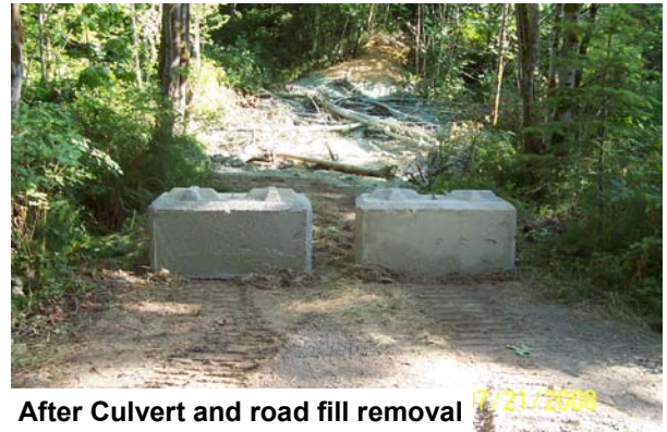
Hannan Culvert Removal Project, Swansonville Cr., FFFPP 06-1685 Stream flowing under road fill. Culvert (undersized) has flow in high water. 3 additional plugged culverts removed during project. At junction SR19 and Swansonville Rd—SE of intersection NW 1/4, S6, T28N, R1E, Jefferson County
