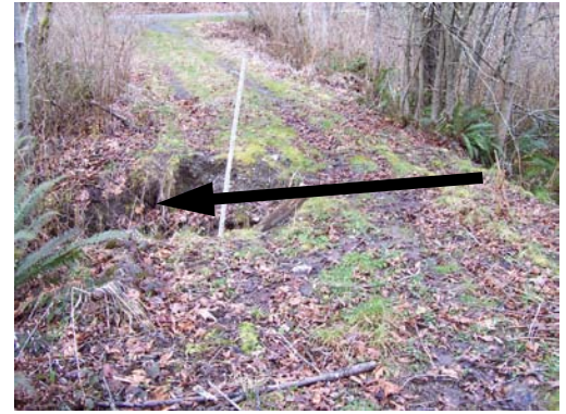
Hannan Culvert Removal Project, Swansonville Cr., FFFPP 06-1685 Stream flowing under road fill. Culvert (undersized) has flow in high water. 3 additional plugged culverts removed during project. At junction SR19 and Swansonville Rd—SE of intersection NW 1/4, S6, T28N, R1E, Jefferson County
