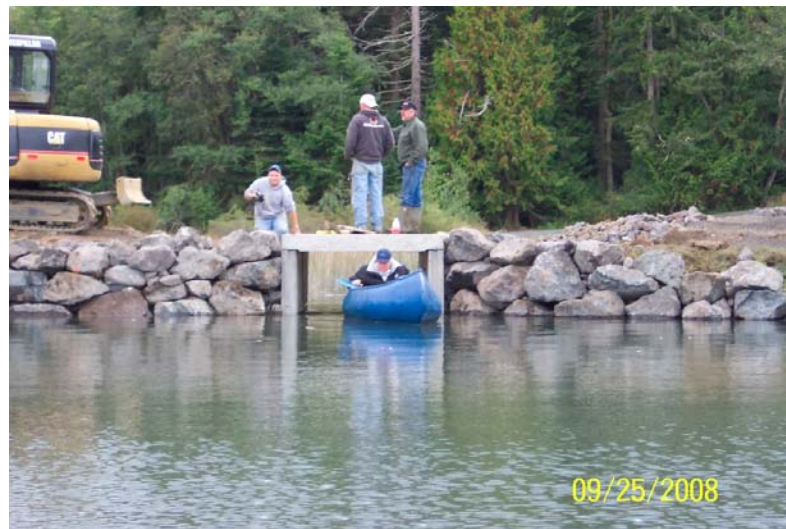
Mystery Bay Culvert Project Summer 2008
