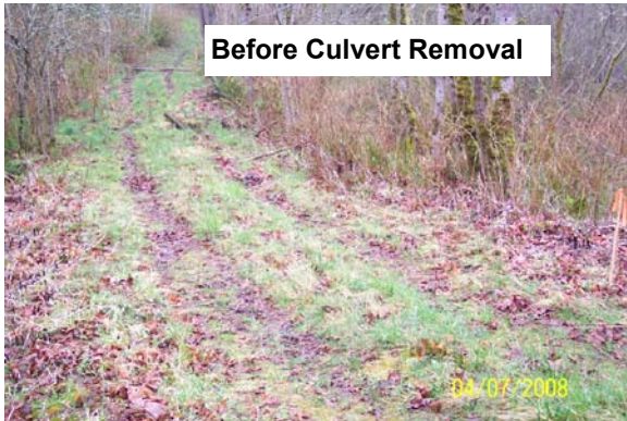
Hannan Culvert Removal Project, Swansonville Cr., FFFPP 06-1685 Stream flowing under road fill. Culvert (undersized) has flow in high water. 3 additional plugged culverts removed during project. At junction SR19 and Swansonville Rd—SE of intersection NW 1/4, S6, T28N, R1E, Jefferson County
