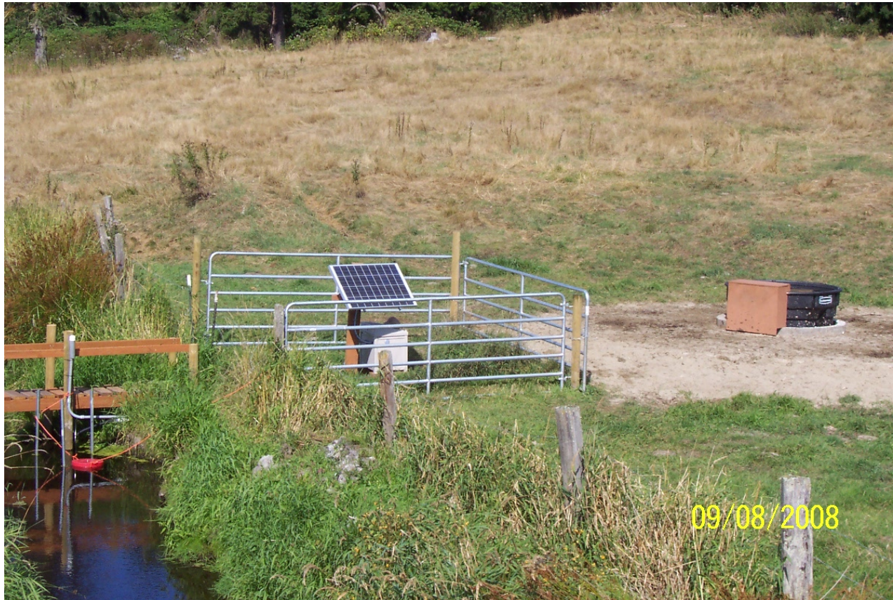
SOLAR POWERED LIVESTOCK WATER SYSTEM Chimacum Watershed
